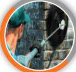
Cleaning Bricks Wall
