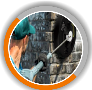
Cleaning Bricks Wall
